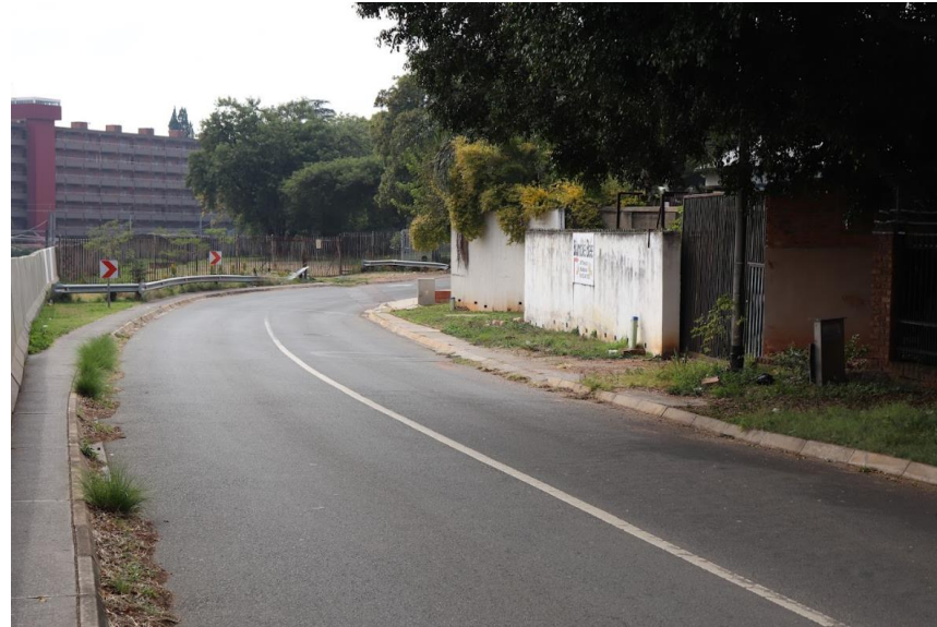
BEREA STREET (EN-ROUTE ELANDSPOORT PARK)
